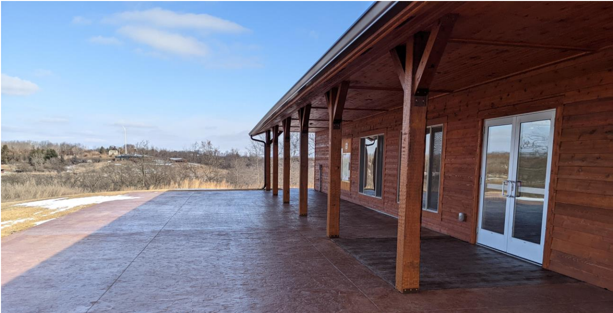
Patio off the West Side of Building
