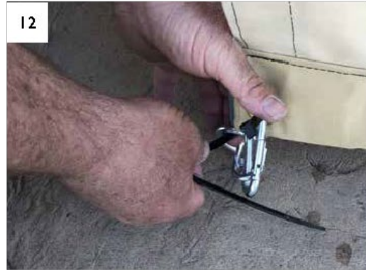
12. Thread the zip tie through the grommet and the eye-bolt.
